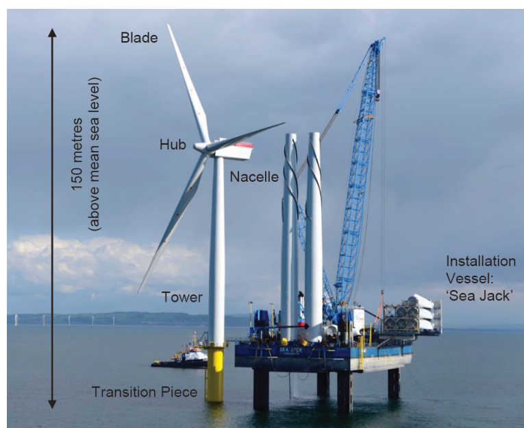
Figure 1.2: Offshore installation of wind turbine [43]
