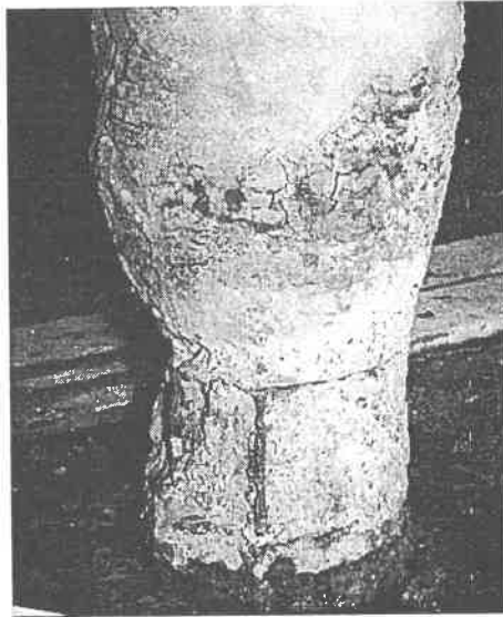
Fig. 14: Arching of green concrete on one of the inner mounting rings. Ring was mounted by welding.
